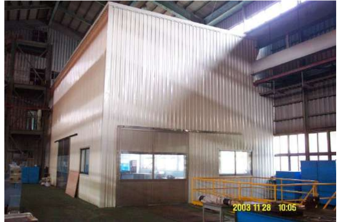
恆溫低污染組裝工作間 Constant temperature clean assembly room
