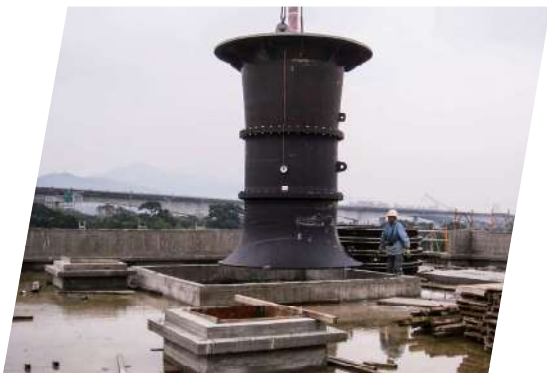
新生擴建抽水站抽水機組 下部組件現場吊裝 Xinsheng pump station On-site installation
