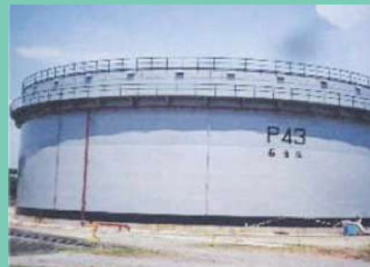
中油 油槽 CPC Oil storage tank
