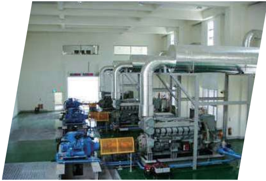
新生擴建抽水站 抽水機組現場安裝 Xinsheng pump station On-site installation
