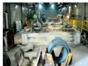
酸洗區 Pickling treatment area
