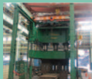
1,500 噸油壓壓床 壓床能力：最大 1,500 噸 1,500ton Hydraulic pressing machine Capacity of pressing force for steel plate : max.1,500 ton
