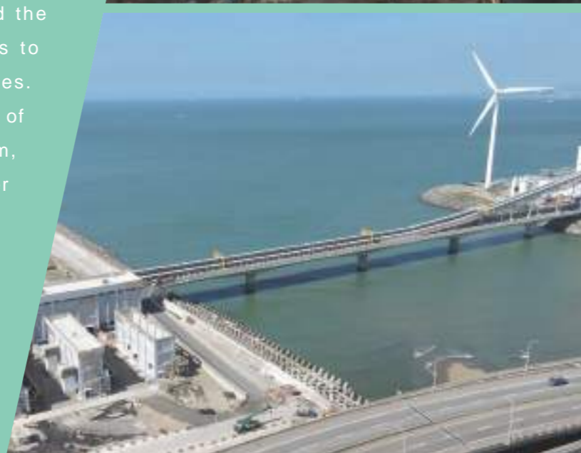
林口電廠輸煤系統 Lin Kou Power Plant Coal Conveying System
