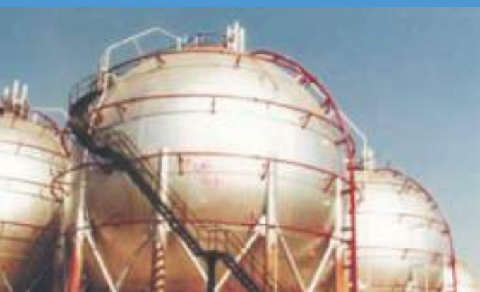
中油 桃煉廠球槽 CPC spherical tank of Taoyuan petroleum refinery
