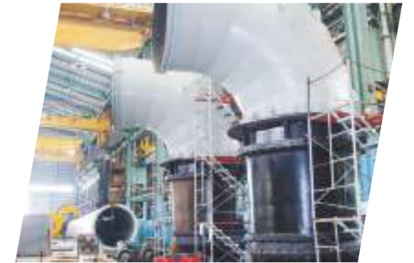
建國抽水擴建站 抽水機於中機廠內組裝 Jianguo pump station Assembling in CSMC
