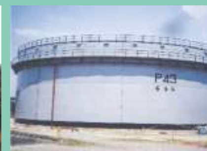
中油 油槽 CPC Oil storage tank
